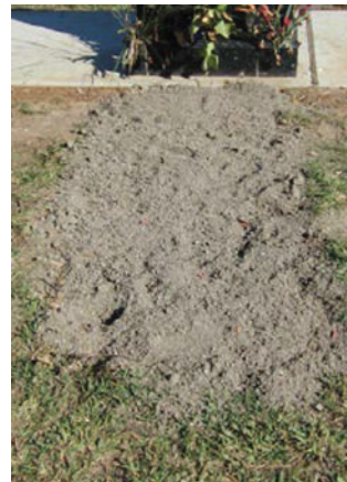
Stabilised grave prepared for turf to be laid
